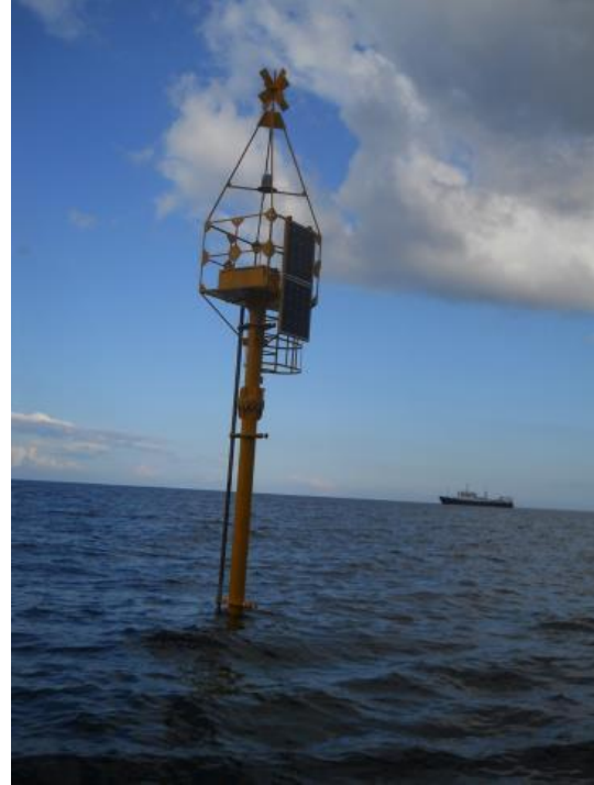
Coastal automatic marine gauge station (Mangalia, Romania)
