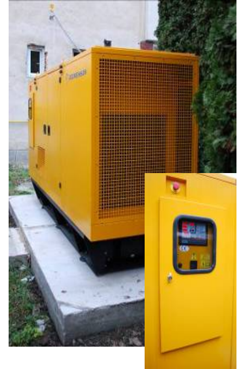
Power generator 275kW
