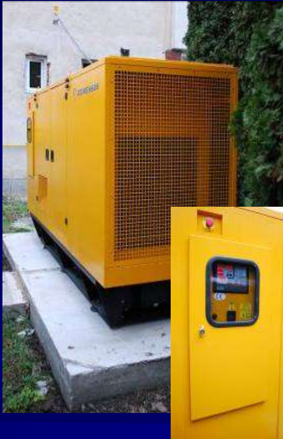
Power generator 275kW
